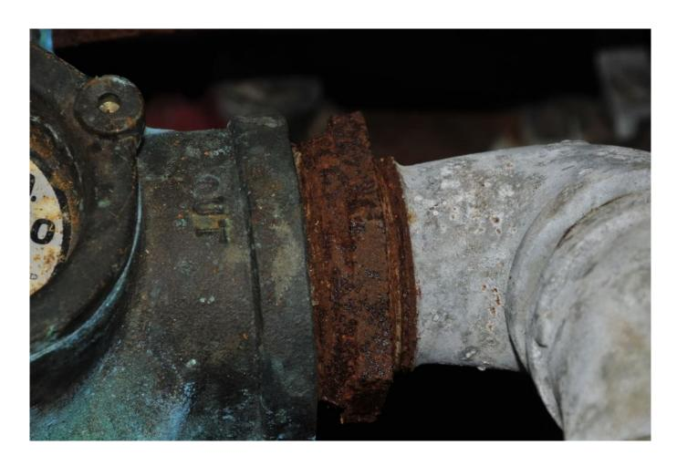
Galvanic corrosion occurs when dissimilar metals are connected and exposed to an electrolyte like seawater. This strainer installation is a textbook example of what not to do, bronze, mild steel and galvanized steel. Not only are these metals incompatible, mild and galvanized steel should not be used for raw water applications.
