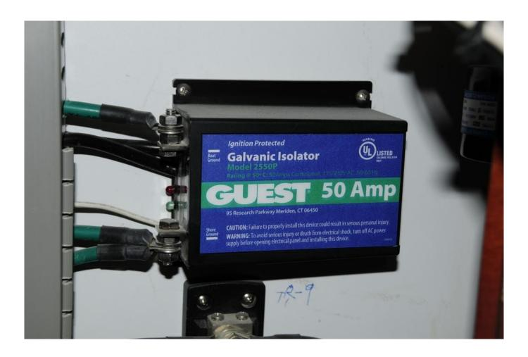
Galvanic isolators are the first line of defense against galvanic corrosion that originates aboard nearby vessels. They are comparatively inexpensive, and easy to install, every vessel equipped with shore power should have one. The one you select should meet ABYC Standard A-28.
