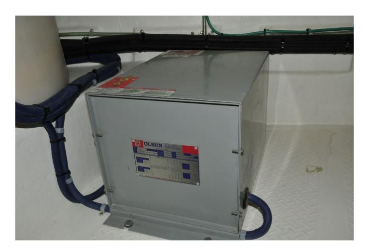
Shore power transformers, when wired in isolation mode, provide an effective and all but impenetrable barrier to corrosion that originates on other vessels, or in places other than aboard the vessel on which they are installed.
