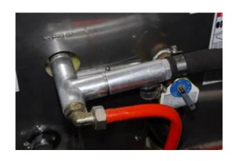
A Temperature Compensating Valve or TCV controls the volume of coolant entering the water heater's heat exchanger, thereby controlling the temperature of the water leaving the water heater.
