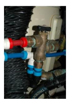
A stock mixing valve, top, that's provided as part of this water heater, along with an aftermarket installation shown on the bottom. Use and adjustment of this device prevents the water heater from supplying water that's too hot, whether it's created by the engine or an electric element.
