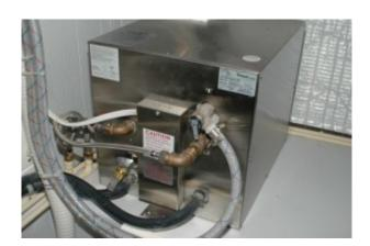
The pressure relief valve is visible in this image, at the upper right corner of the water heater case. Note the attached red and blue trace extension hose.
