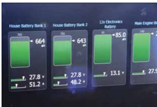
The monitor’s central readout permits at-a-glance observations for a range of systems, and allows the operator to set and adjust alarms for voltage, temperature, pressure, and levels.
