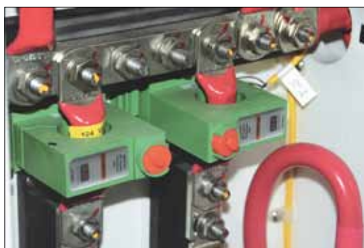
Above —The integrated vessel-monitoring system from Krill Systems (Bainbridge Island, Washington) allows the operator to monitor a wide variety of gear, from electrical and hydraulic systems to tankage and temperatures. Left —Krill Systems current transducers monitor electrical flow in multiple locations throughout the system.
