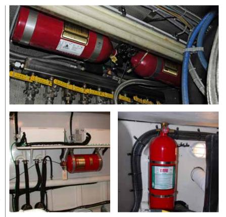
A fire extinguising system must be capable of flooding the space it protects. Combining two smaller bottles (top) would not comply with standards unless each could flood the space. Tanks should be mounted as high as possible in the engine room and away from ventilation systems (above, left). Installing the bottle's heat-sensitive nozzle close to the overhead enures it will trigger quickly in case of a fire.
