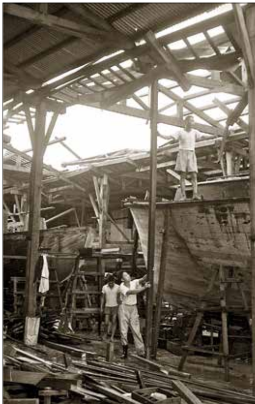
Crews inspect and shore up the American Marine boatbuilding facility in Junk Bay, Hong Kong, in the aftermath of Super Typhoon Wanda, which hit September 1, 1962, just three months after Fleming began overseeing engineering for the yard.
