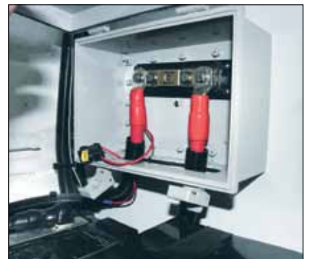
Left —Two parallel series strings of two batteries each allow for high amp-hour capacity at the desired 12V-system voltage. Above —Over-current protection of large battery banks is a critical requirement. Class T fuses are well suited for this role. The fuse shown here is an ANL, which lacks the appropriate ampere interrupt capacity for the large bank it serves.
