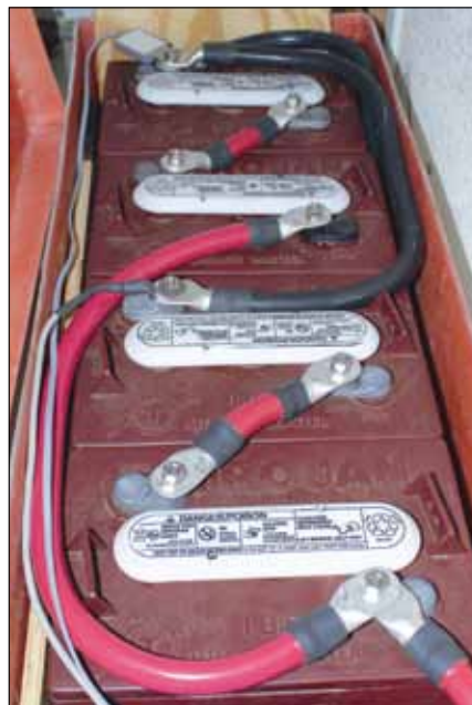
Left —Two parallel series strings of two batteries each allow for high amp-hour capacity at the desired 12V-system voltage. Above —Over-current protection of large battery banks is a critical requirement. Class T fuses are well suited for this role. The fuse shown here is an ANL, which lacks the appropriate ampere interrupt capacity for the large bank it serves.
