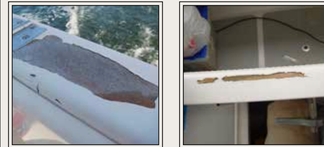
Though durable, even two-part coatings have their limitations. On this teak rail (left), the wood's tendency to expand and contract with changes in humidity and temperature, along with its natural oils, make adhesion challenging. The edge of this timber hatch (right) has been abraded by the hatch frame, allowing water to enter, which in turn has caused the paint to lift.
