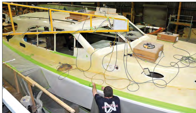
A PB 50 in construction. The drive for perfection shows in the company's emphasis on hull finish, particularly at the tumblehome in the stern quarters, because “it’s the part of the boat people look at most,” said Richards.
