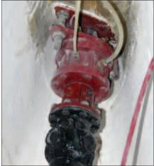
**Top**—The signage posted above the zerk fitting is mistaken: thrust bearings do require greasing, but most don't require it very often. To avoid over-greasing, follow the equipment manufacturer's guidelines. **Above**—Here, instead of grease lubrication, an oil reservoir gravity-feeds oil to the thrust-bearing assembly.
