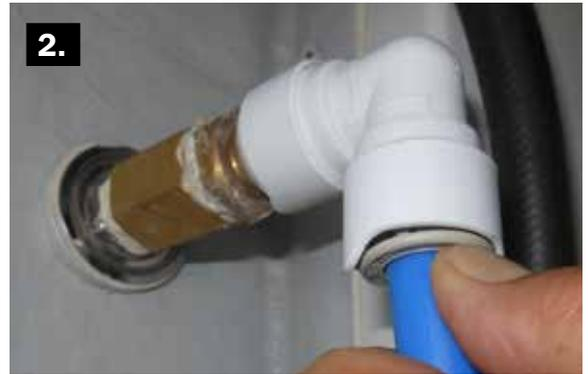
**1.** Reliable, easy-to-install proprietary plumbing systems commonly employ PVC tubing, **1**, and PEX tubing, **2**. Those that rely on O-rings for watertight seals are prone to leakage when stressed or if tubing and receivers don't remain parallel. **3**—To eliminate the stresses that could cause leaks, accessory fittings hold the tubing in a gentle 90° curve as they enter the manifold.
