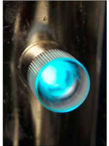
chamber illuminated with a UV light, which kills most biological life-forms. Provided it's sized properly and maintained (the bulbs require periodic replacement, often annually), this is yet another effective step to ensure that water is clean and contaminant-
