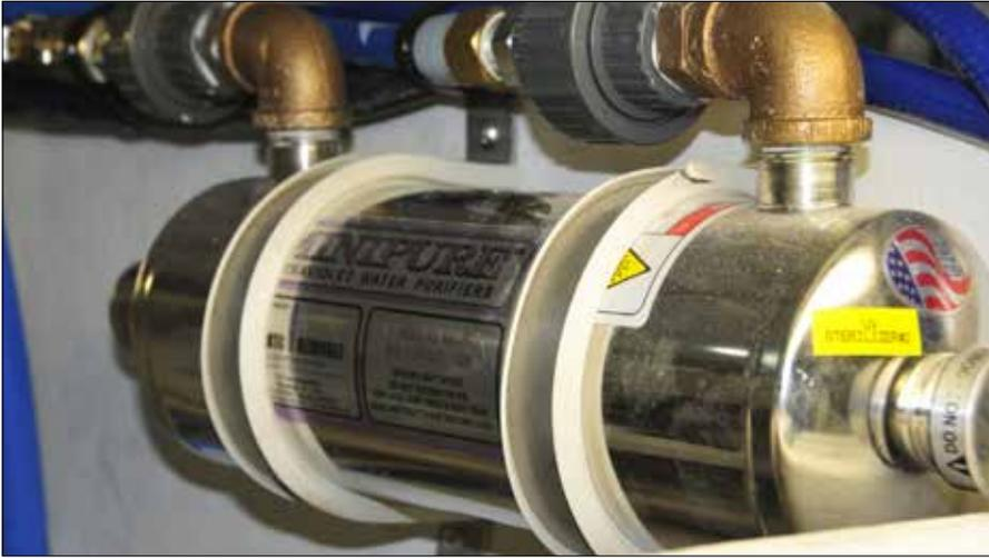
*Water-treatment systems that rely on ultraviolet light are effective at eradicating biological contamination. Most include a sight glass to confirm operation of the bulb. When installing these filters, ensure access for bulb replacement.*
