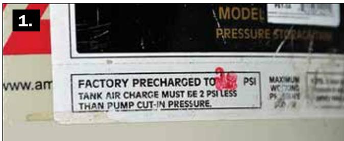
**1**—Accumulator tanks are typically pre-charged with a head of air (this one rated at 28 psi), which reduces the “water hammer” effect and pump short-cycling. **2**—Reliable self-priming DC diaphragm pumps can eliminate the need for an accumulator tank in smaller systems. **3**—Larger vessels rely on 120 or 240VAC non-self-priming pumps. This model is equipped with a proprietary pre-filter to prevent debris from damaging the pump.
