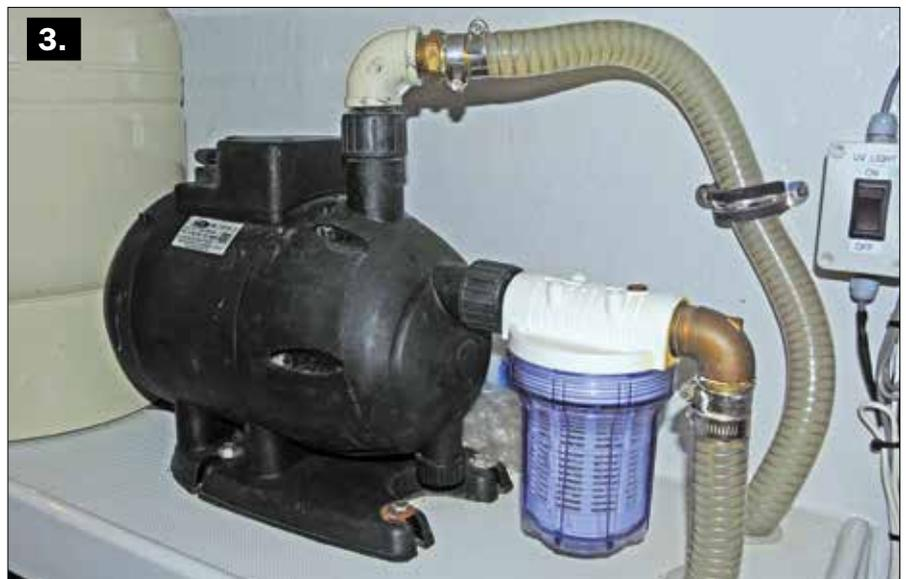
increases, so does the speed of the pump's motor. The result is smoother, more consistent flow without the need for an accumulator tank.
