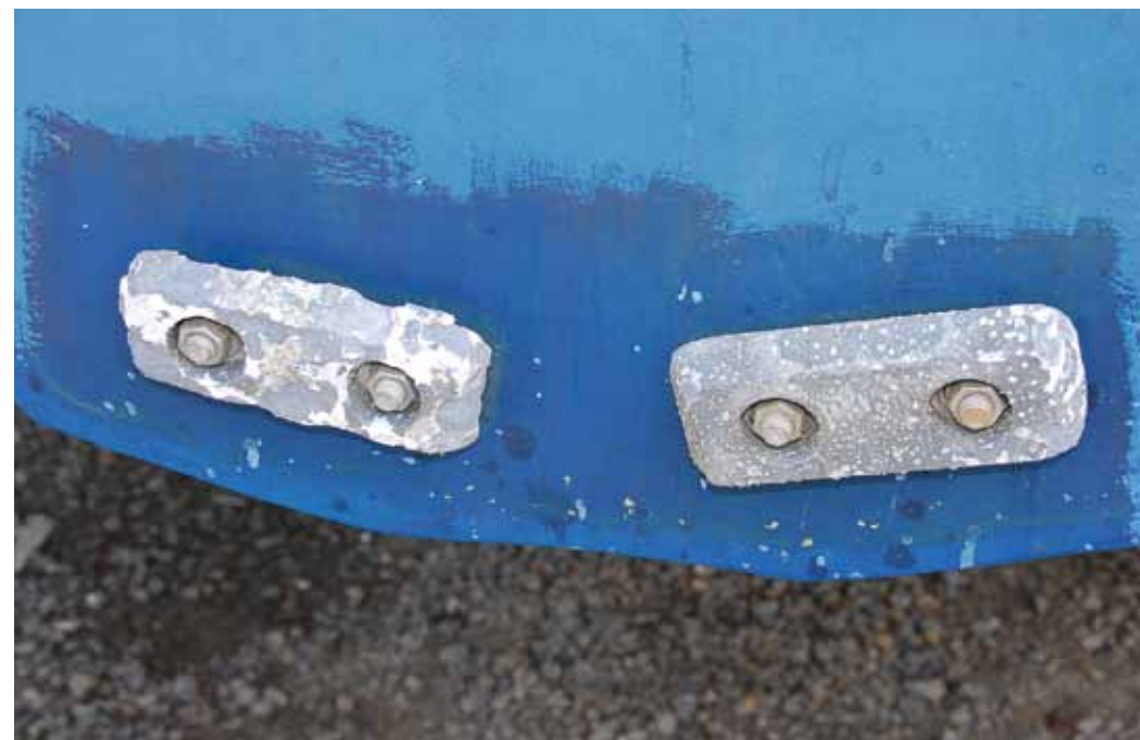
Anodes should decay at roughly the same rate, especially those that are the same size and collocated, when one remains near pristine it's usually a sign of a poor bonding system connection.
