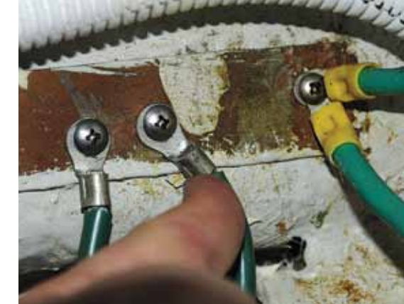
Bonding connections must offer a low resistance electrical path, which means they must be tight and free of corrosion.
