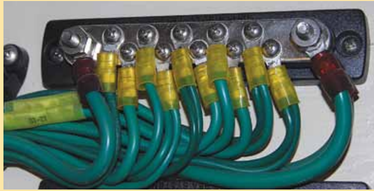
Bus bars are an effective, low resistance means of connecting multiple bonding system wiring runs.
