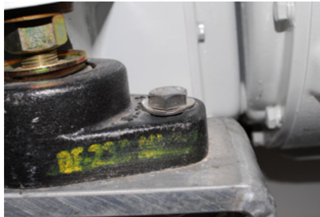
Washers used with all motor mount hardware must be resistant to distortion.
