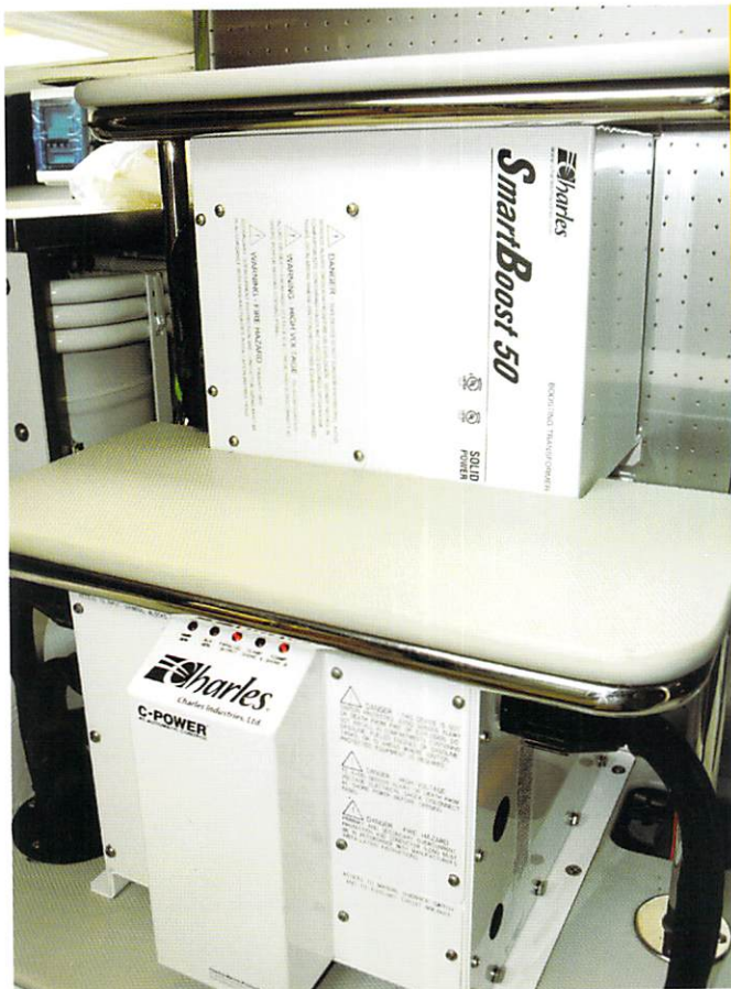
F55 Shorepower equipment, includes voltage boost feature
