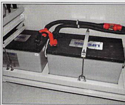
Battery boxes are especially well-suited to flooded battery installations (left); however, the shoebox-like lid must not form an envelope in which hydrogen gas can be captured. Batteries must be secure and completely immobilized, and their positive terminals must be insulated. This installation (center) covers all those bases. A fiddle or frame around a battery bank (right) can serve two purposes: to contain electrolyte and to keep the batteries stable.
