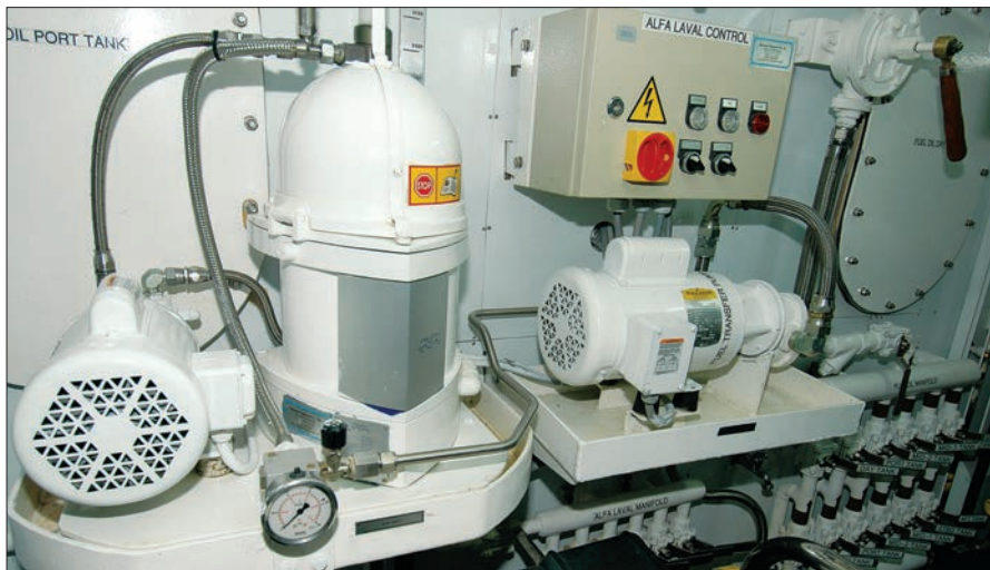
An Alfa Laval separator—installed aboard a 65'/19.8m motor yacht—is plumbed via a manifold to each of the vessel's tanks, and polishes fuel before any is pumped to a day tank.
