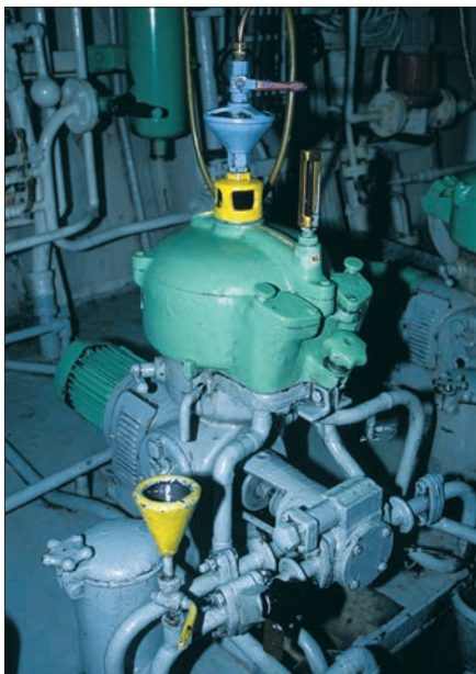
A 40-year-old centrifugal separator . It's still going strong aboard an expedition cruise ship that operates from Arctic to Antarctic waters, where fuel filtration is critical but the nearest spare filter-element may be thousands of miles away.
