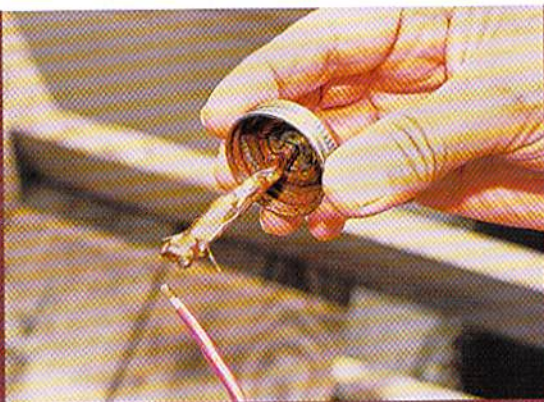
Copper conductant paste being applied to a conductor prior to crimp installation. This makes for a durable, trouble free crimp that will last for many years.
