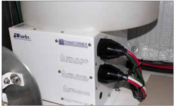
Left —One of the most common transformer installation faults involves inadequate chafe protection and strain relief where wires pass through the metal housing. Right —This approach, using nonmetallic compression fittings, is ideal.
