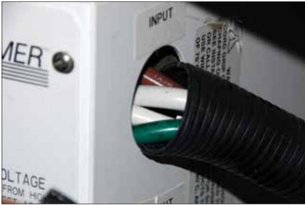
Left —One of the most common transformer installation faults involves inadequate chafe protection and strain relief where wires pass through the metal housing. Right —This approach, using nonmetallic compression fittings, is ideal.
