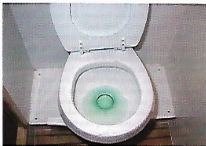
Winterizing sanitation systems calls for the removal or displacement of all raw water from plumbing and fixtures. For freshwater flushing systems, such as the vacuum toilet shown here, the freshwater plumbing also must be flushed with nontox.
