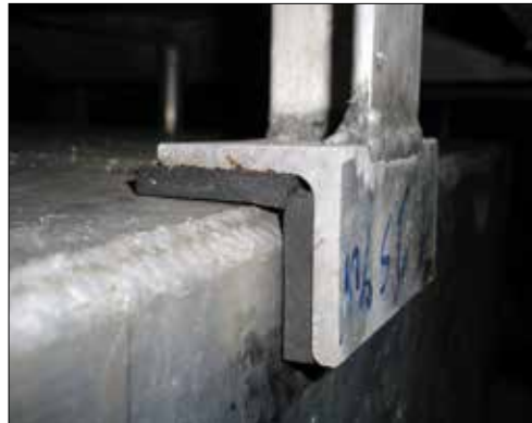
Left —Integral flanges are an ideal means of securing a tank. Note the shim slightly elevating the tank from the supporting shelf.
