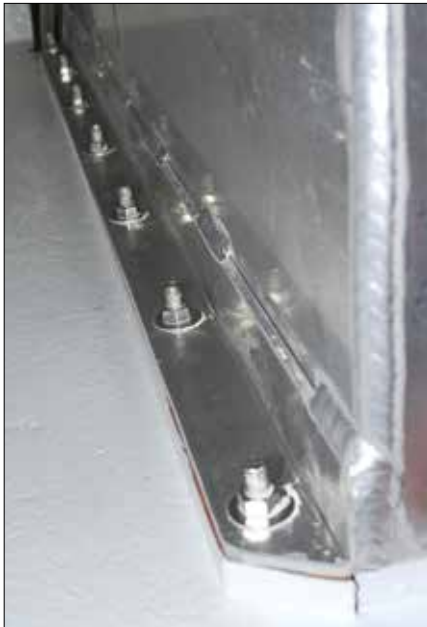
Left —Integral flanges are an ideal means of securing a tank. Note the shim slightly elevating the tank from the supporting shelf.
