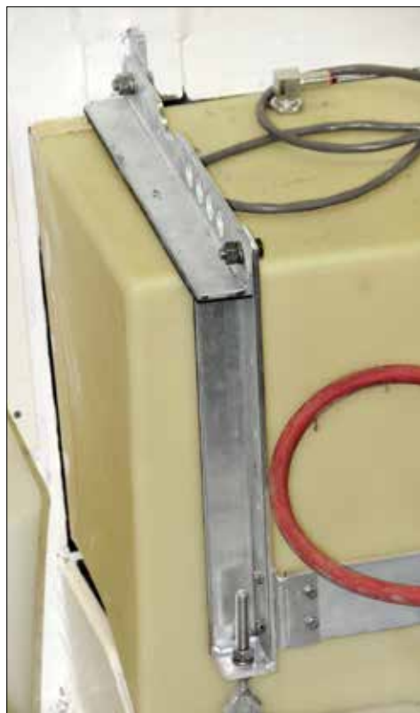
Left —This poly tank is supported with substantial aluminum cribbing. Note the threaded, adjustable attachment post at the lower corner.
