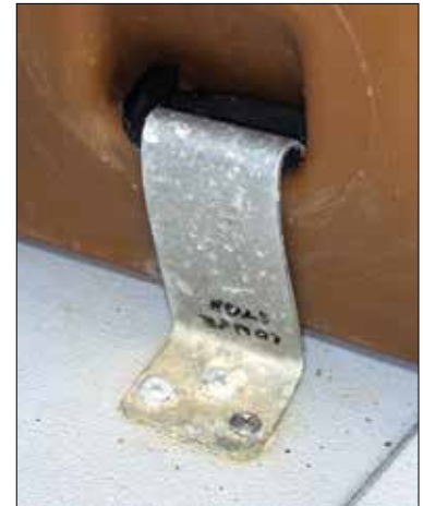
Above —This metal tank is supported from above, but the cushion material is not bonded to the tank, which means it can trap water, leading to corrosion. Right —While a claw retainer fits the molded recesses of this tank, it is corroding. Also, even when new the small tapping screws securing it aren't adequate to resist the loads of the full tank.
