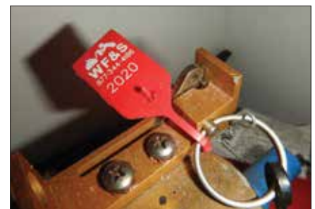
Left—Mount the bottle as high as possible in the compartment. Below—The safety or shipping pin prevents unintentional discharge during installation and maintenance but must be removed when the system is in service.
