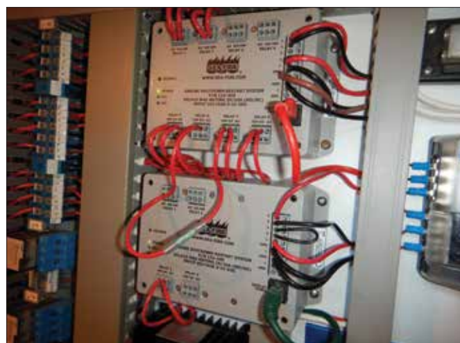
A connected relay kit automatically shuts down circuits for engines, generators, and blowers and activates ventilation shutters when the system is deployed.
