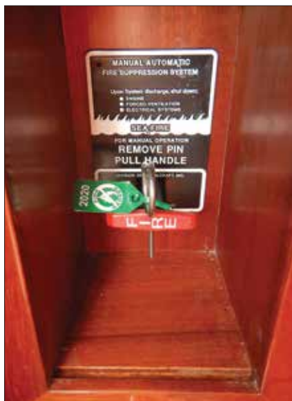
Left—The manual-discharge T-handle should be secured with a safety pin and breakaway plastic tie. Below left—This helm display has an audible alarm and red and green lights to indicate when the system is charged or discharged (both illuminated here during a test).
