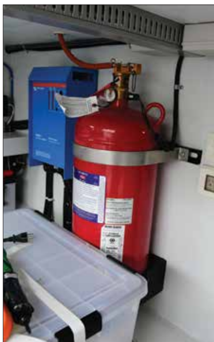
Left—Mount the bottle as high as possible in the compartment. Below—The safety or shipping pin prevents unintentional discharge during installation and maintenance but must be removed when the system is in service.
