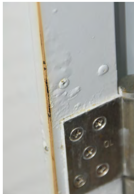
Left—Corners of metal structures are often subject to excessive abrasion and frequently suffer from thin paint coverage making them particularly vulnerable to corrosion. Right—Especially on aluminum spars, paint failures tend to propagate from hardware installations.
