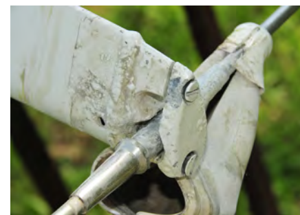
Aluminum sailing rig hardware kept in a moist environment under the rubber spreader boots is particularly vulnerable to corrosion.
