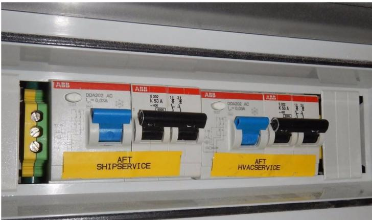
**ELCI's, the blue-handles, are often combined or co-located with primary shore power inlet circuit breakers, the black two pole devices to the right of the ELCI. Don't assume an ELCI trip current is correct, as they are available in a wide range, from 5 mA through 100 mA. ABYC compliant ELCI's should be designed to trip at 30 mA, those seen here indicate this in the ?I=0,03A? shown on their face.**
