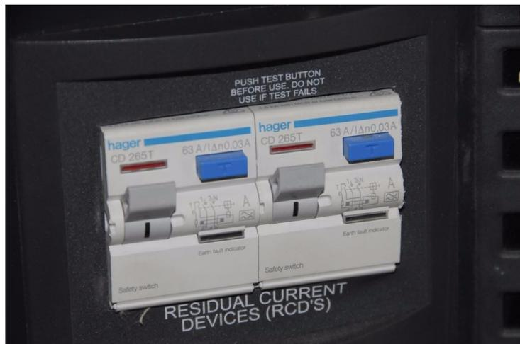
**Like GFI's, ELCI's (sometimes referred to as RCDs) must include a test feature, the blue button with embossed T.**
