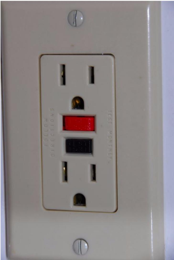
**Ground fault interrupter receptacles have been around since the 60's. Having saved countless lives in that time, they should be installed in a vessel's head, galley, on weather decks and in engine rooms and machinery spaces. They provide local protection and are still required even for vessels equipped with an ELCI.**
