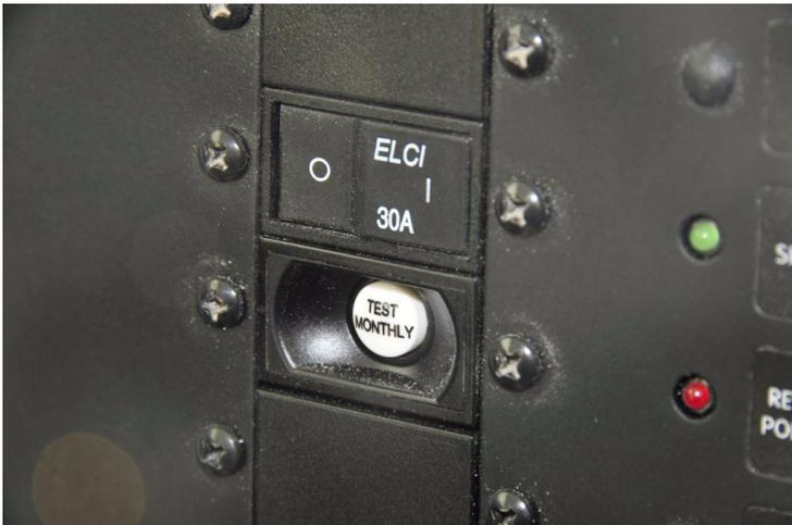
**If the wire-run distance between the shore inlet and the circuit breaker panel is less than 10 feet, the ELCI may be located in the latter.**
